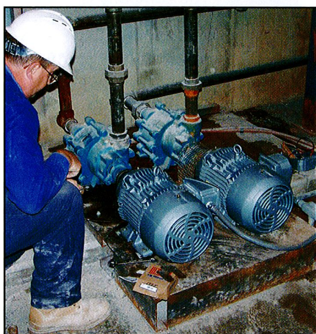
Figure 4. An electrician installs two new copper-rotor 10-hp SE&A IEEE Plus motors that will supply boiler feedwater for process steam. The SE&A motors are rated for a NEMA nominal efficiency of 92.4% at 100% load factor, which exceeds the NEMA Premium requirement by 0.7 percentage points. Tests conducted for CDA show that a copper-rotor SE&A motor of this size actually displays an efficiency of 92.72% at full load and greater than 93% at a 75% load factor.
