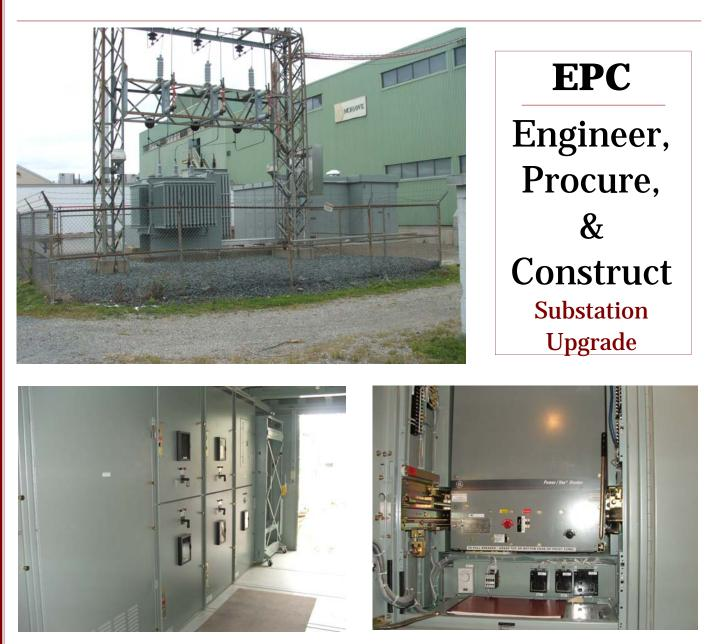
A paper mill in Cohoes, NY was in need of a primary substation upgrade. The exisiting 3750KVA primary substation transformer servicing the facility had reached it's maximum capacity and the existing secondary 5KV main breaker was feeding a bank of (4) 5KV load break switches.
